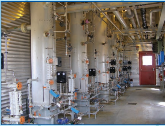
Enhance safety by scanning overhead piping from ground level.
